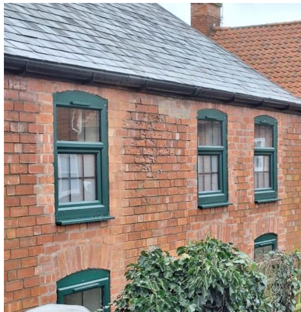
Site photo showing the replacement windows.
