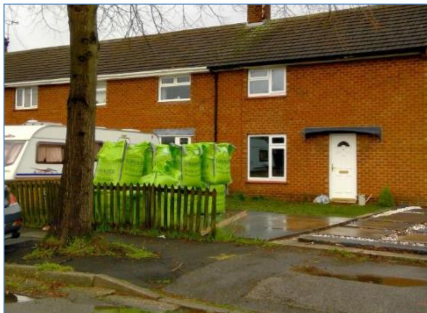
Site photo showing the site following the removal of the unauthorised development.
