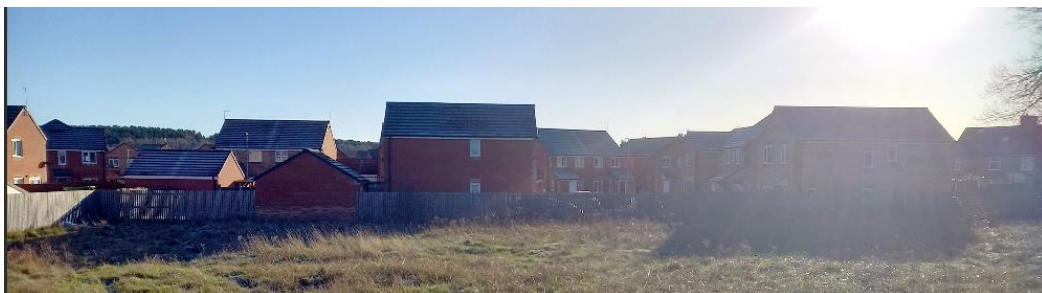
Side of recently constructed dwellings to the south of the site
